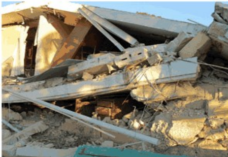
After the earthquake at the school in Riviere Froide
